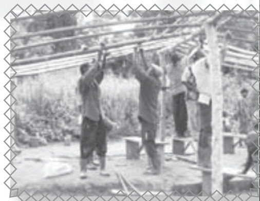
Putting up the roof supports.
