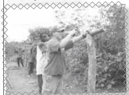
Andy helping build the Satikran church walls.
